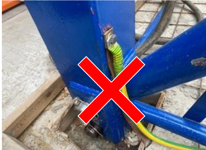
Figure 2: Earth incorrectly connected to a non-manufacturer approved point. The structural member should not have been drilled and tapped as this could weaken the member.
