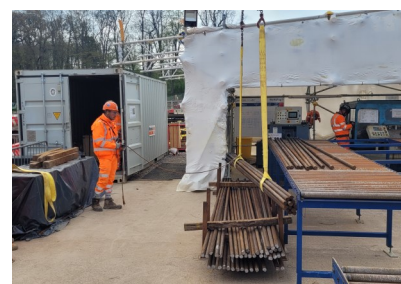
Direct load control necessary. SS using tagline for safe positioning.
