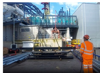
No requirement for direct load control. SS stood away from the load.
