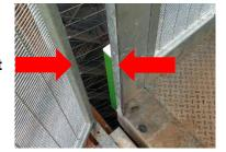
The hoist, designed for up to 10 persons is fully enclosed, but the gap allows for the movement and safe operation of the lift.
