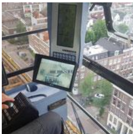
Figure 5: Monitor in operator cab
