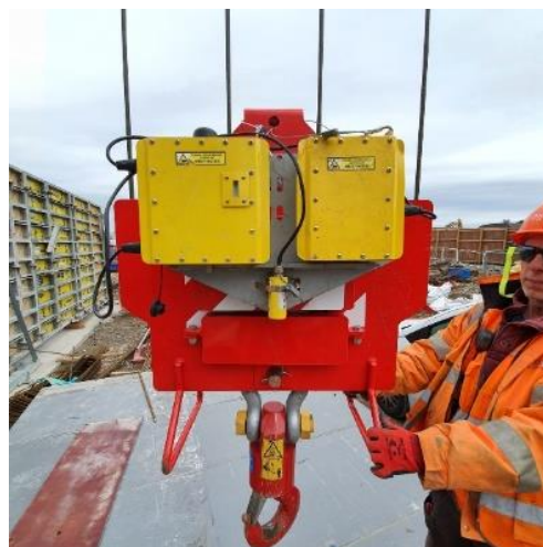
Figure 3: Inspection of hook mounted camera by slinger whilst hook block is at ground level
