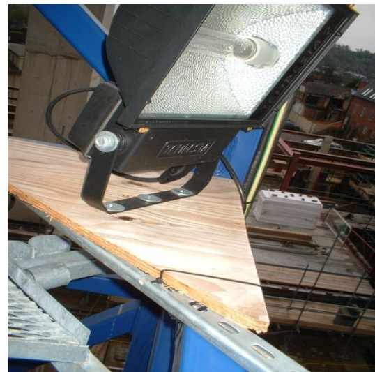
Figure 2 - Unsafe Fixing
