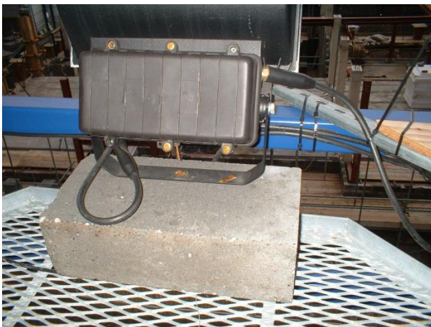
Figure 1 – Unsafe Fixing
