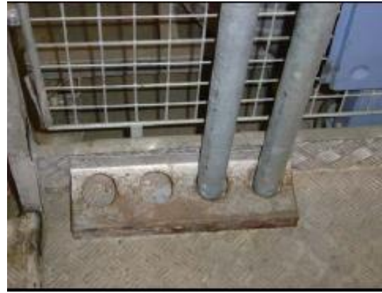
Examples of Scaffold Tubes Held Securely Top and Bottom
