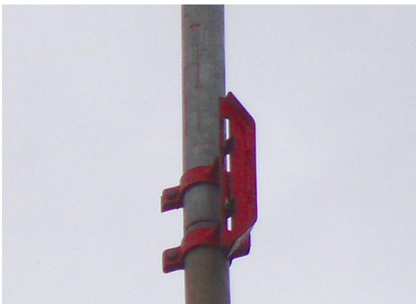
Figure 2 - Temporary Cage Gate Interlock Ramp for a Passenger Hoist Based TSTS
