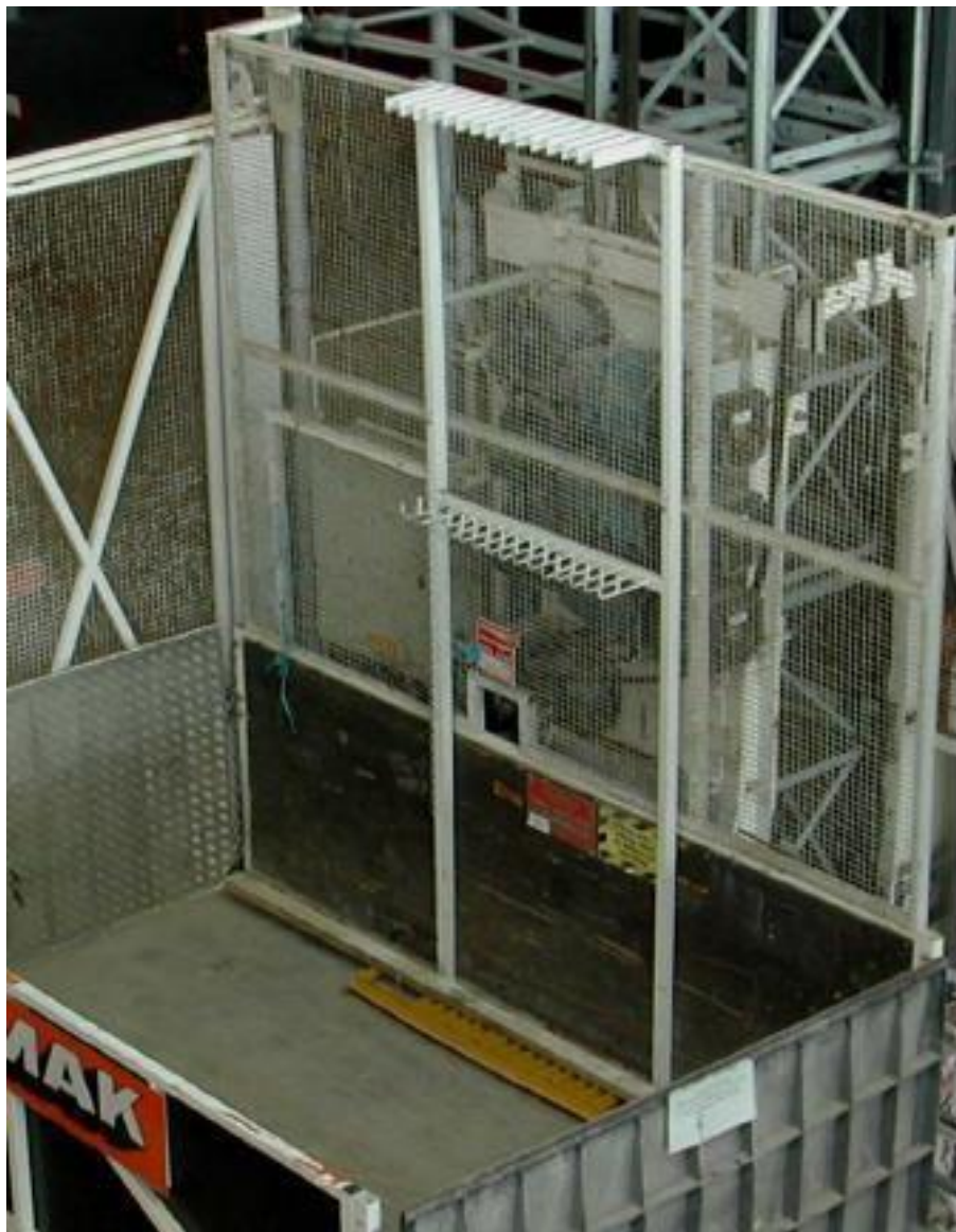
Tube Rack on the Platform of a Goods Only Hoist
