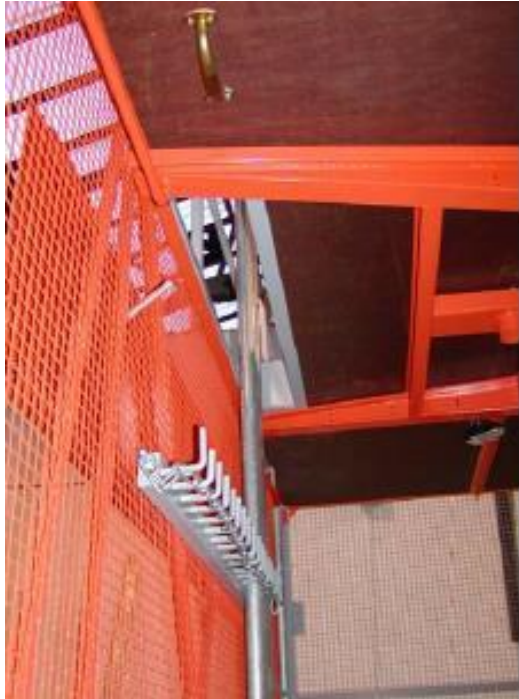
Scaffold Tubes Secured at Floor Level and by a Rack on the Wall
