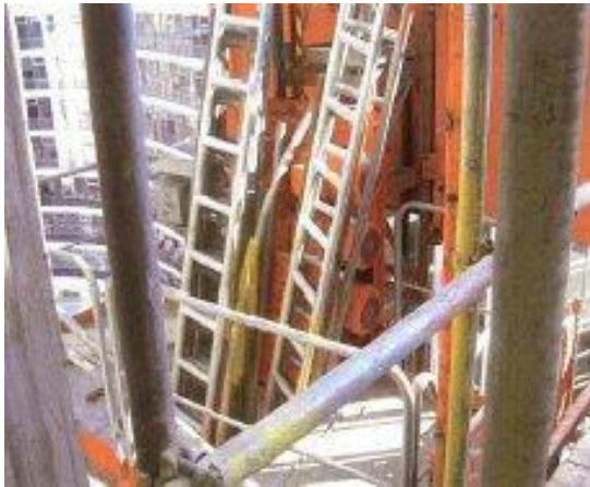
Unsecured scaffold tube jammed in mast.
