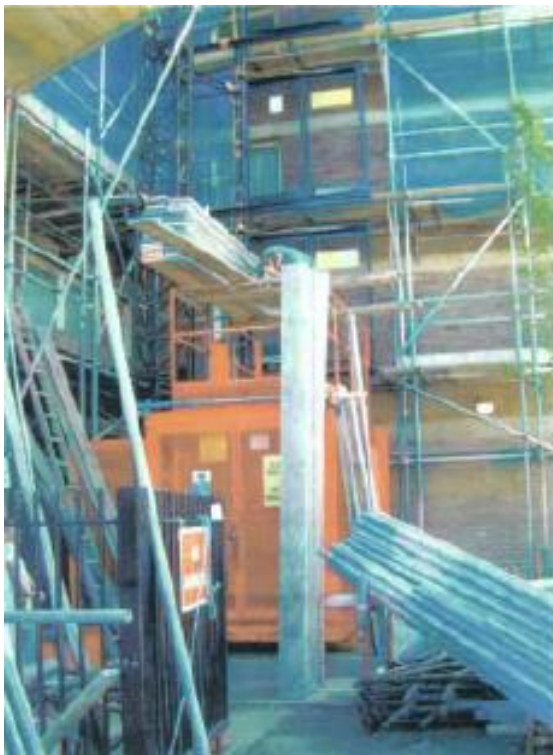
Never load materials on handrails. Handrails are not designed to take high loads and may collapse causing the materials to fall.
