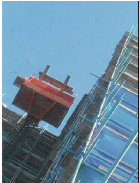
Never allow materials to project outside the confines of the cage/platform. The overhanging materials may catch on a projection into the hoistway and fall onto people below.
