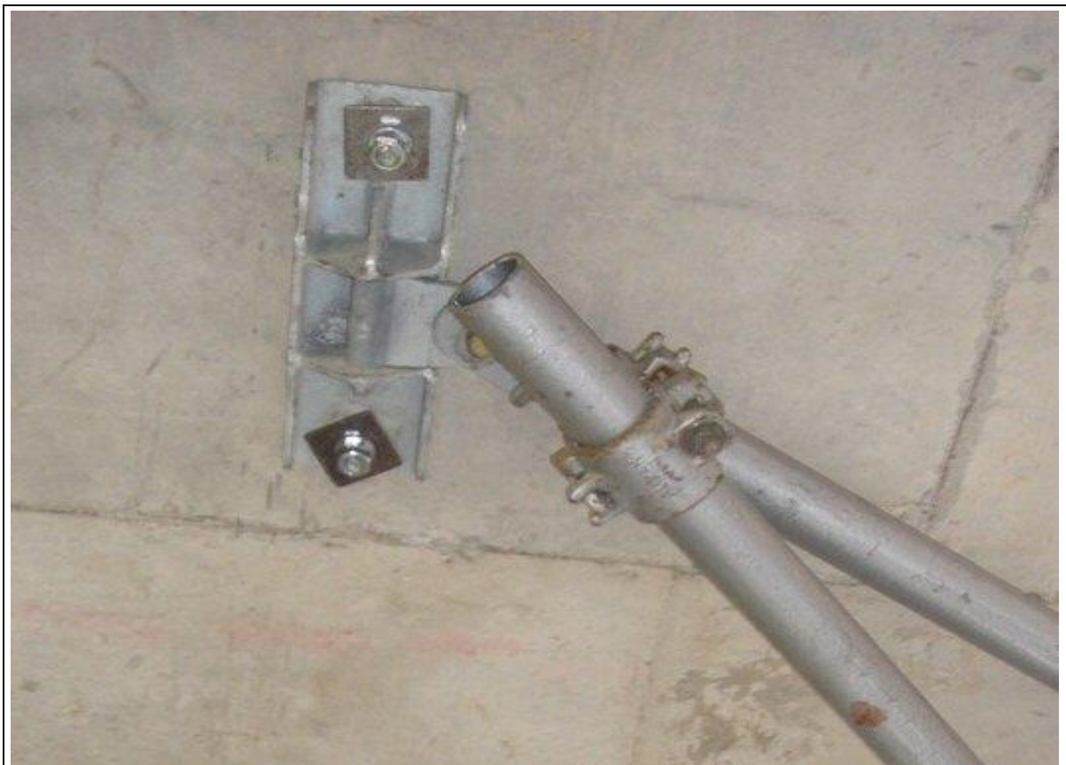
Figure 8 – Tie to Underside of Concrete Slab
