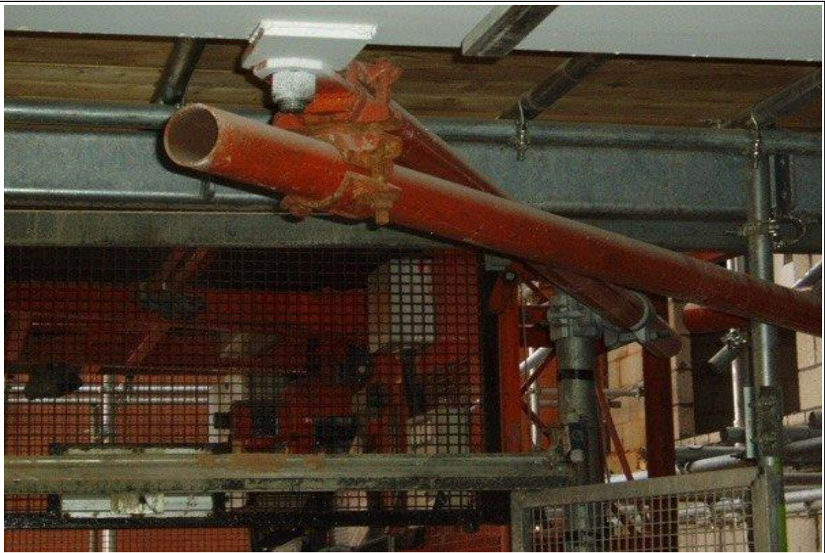
Figure 9 – Tie to Steel Structure
