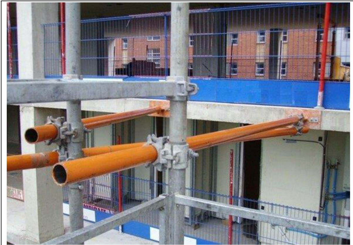
Figure 7 – Tie to edge of Post Tensioned Concrete Slab
