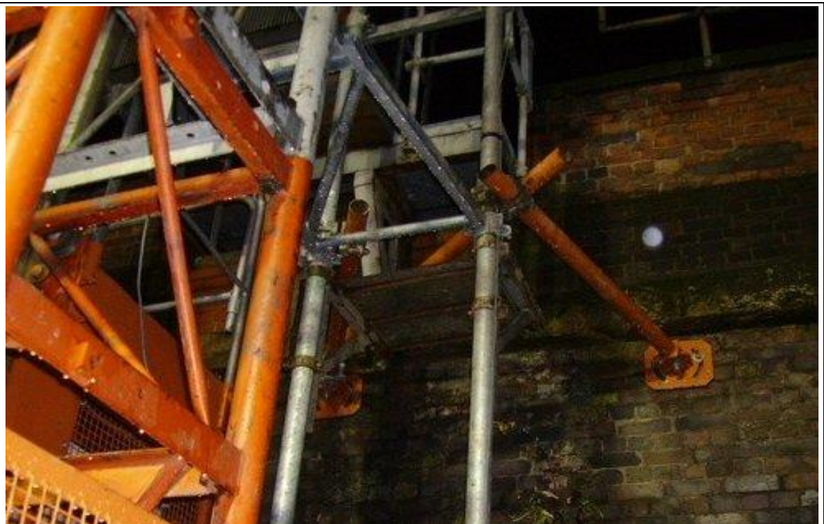
Figure 10 – Tie to Brickwork
