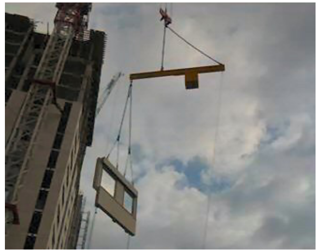
Figure 1 - Use of a Cantilever Lifting Beam
