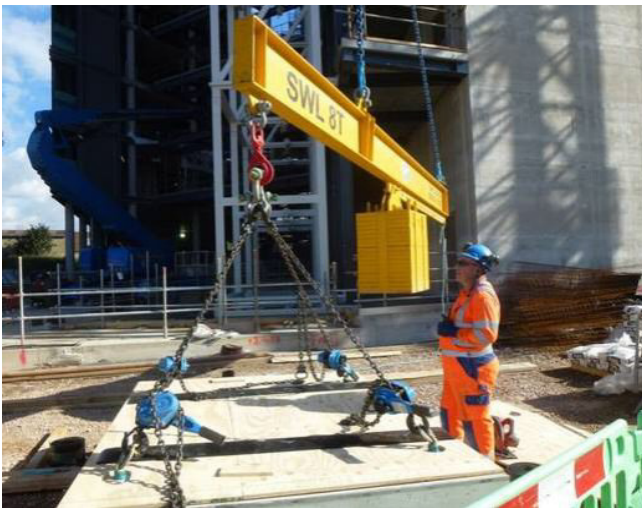
Figure 1 - Use of a Cantilever Lifting Beam
