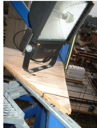
Figure 2 - Unsafe Fixing
