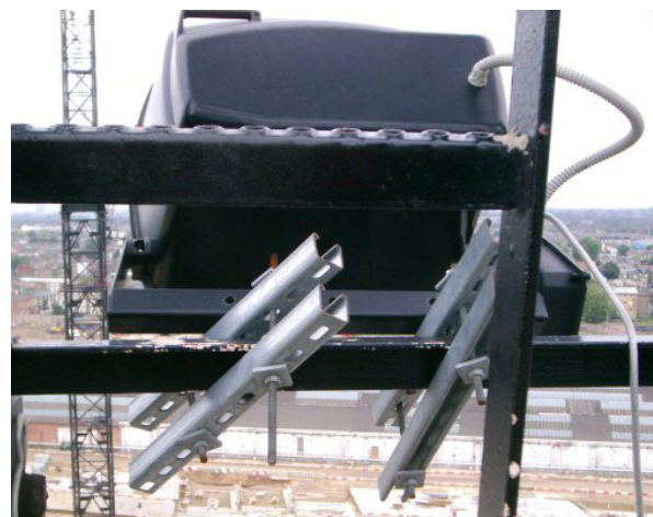
Figure 4 - Safe Fixing
