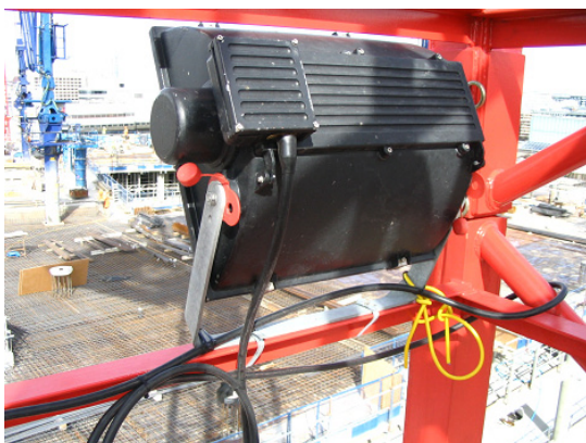
Figure 3 – Unsafe Fixing
