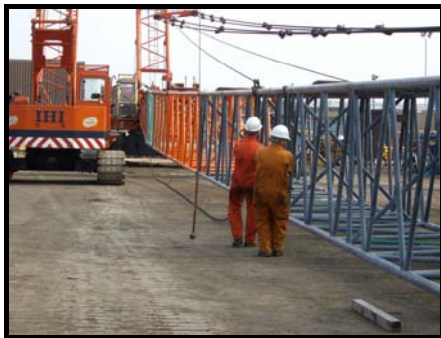
Fig. 3 – Extending Rope At Ground Level
