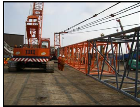
Fig. 2 – Extending Rope At Ground Level
