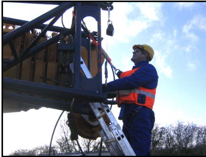
Figure 2 - Work Positioning System
