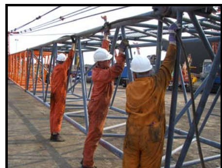
Fig. 6 – Lifting Rope Onto Jib
