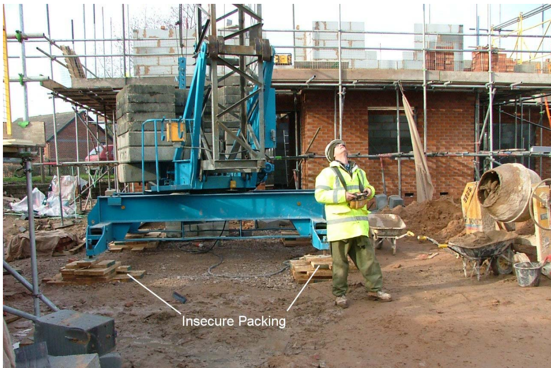
Insecure packing under outriggers (See 5.3)
