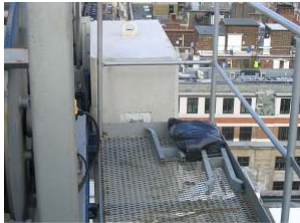
Figure 2 – Poorly Stored Components
